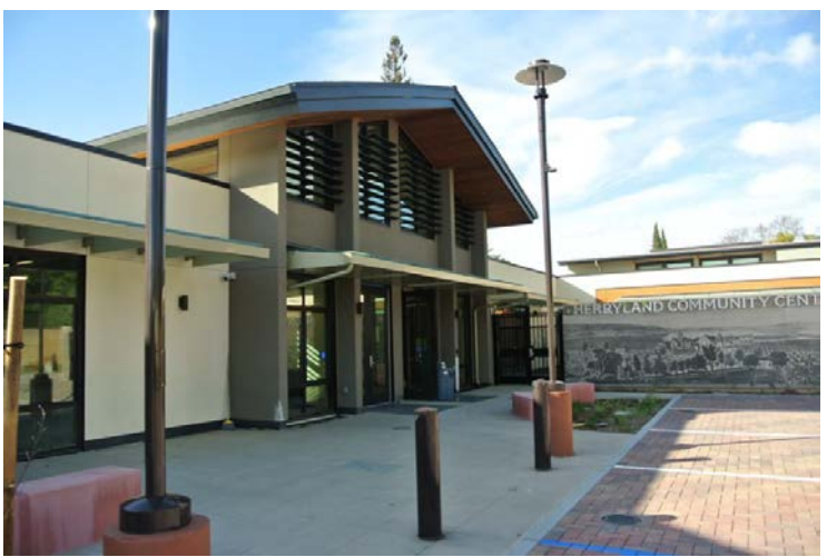
The new Cherryland Community Center was built in partnership with the Hayward Area Recreation and Park District (HARD), who will operate this new community resource.
